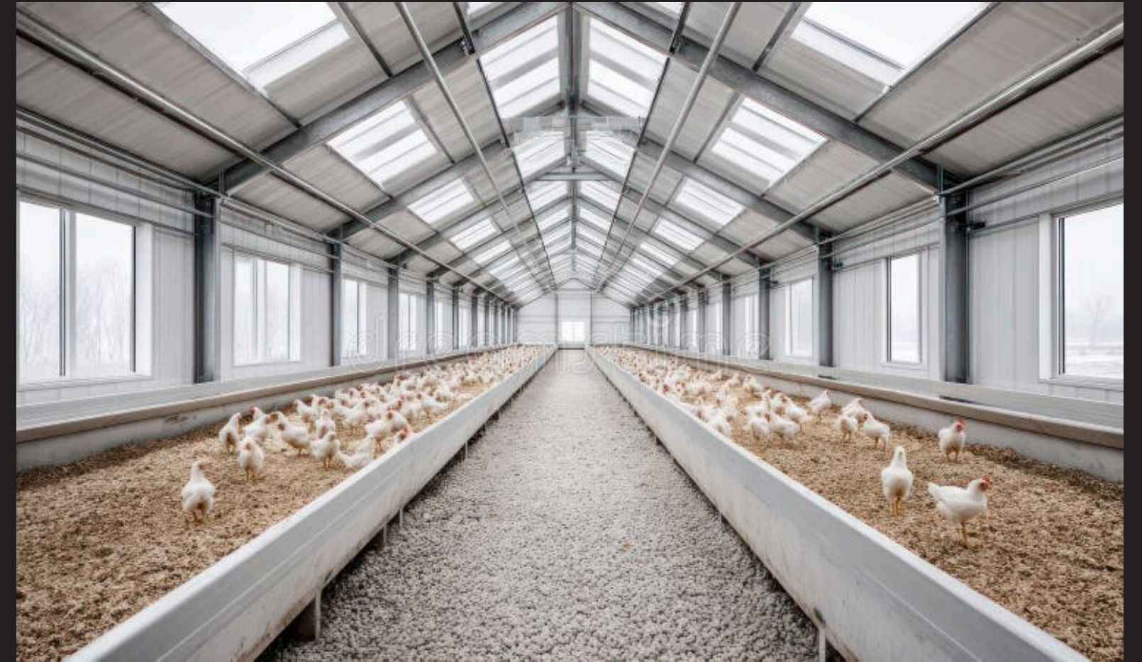
Modern poultry production facility
